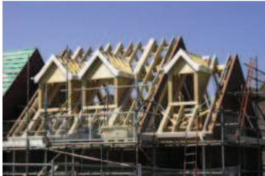
Figure 4 In 2014 Barratts began building 41 additional homes in Bishop Sutton
